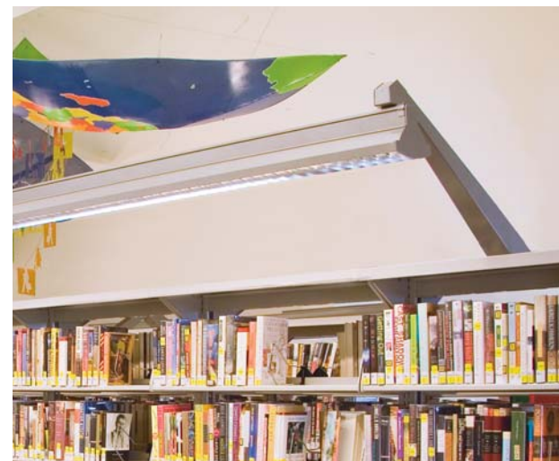
Matching one-way arms support stacklights along the first and last faces of shelving.
