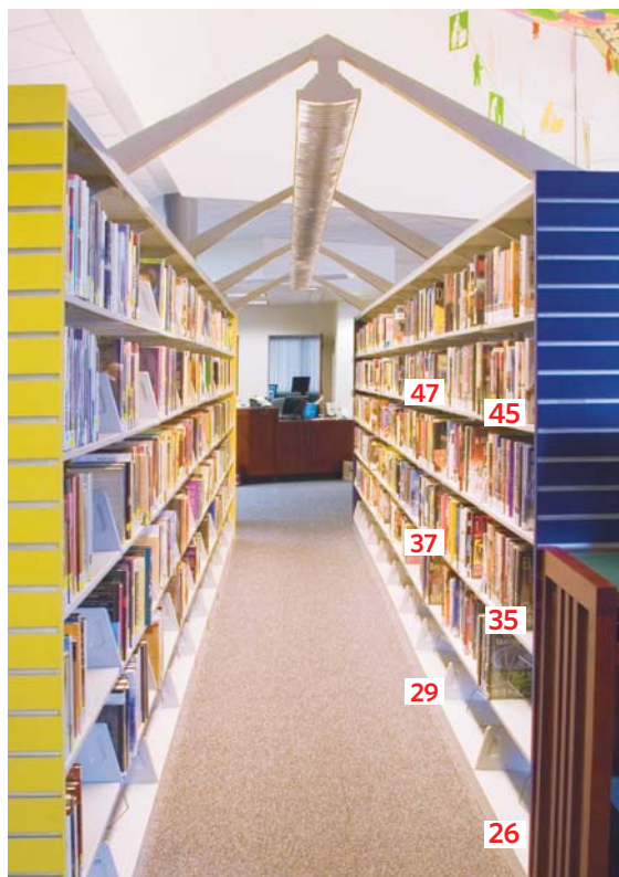
Vertical fc levels at 6", 30" and 54" above floor, measured mid-length and 4' from end of aisle after 500 hours of operation.
